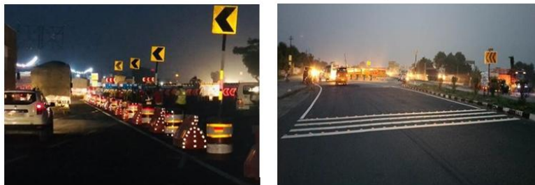
Road Diversion in the night
